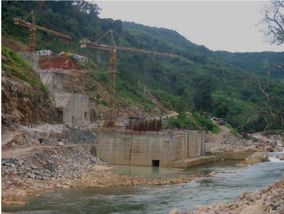
A BIRD EYE VIEW OF THE DAM UNDER CONSTRUCTION
