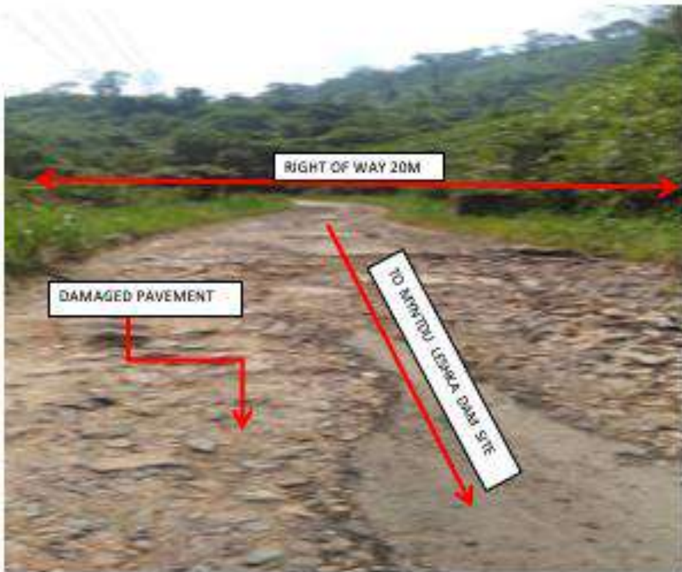
Figure 1.2: Current Status of Approach Road with Width of its ROW
