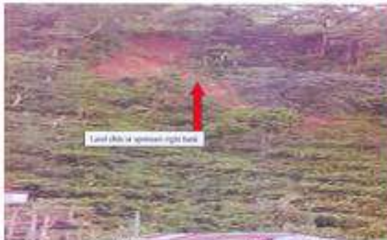
Landslide at upstream Right Bank
