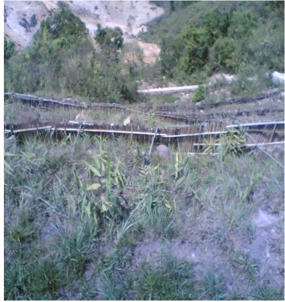
Bamboo pallasiding and Turfing
