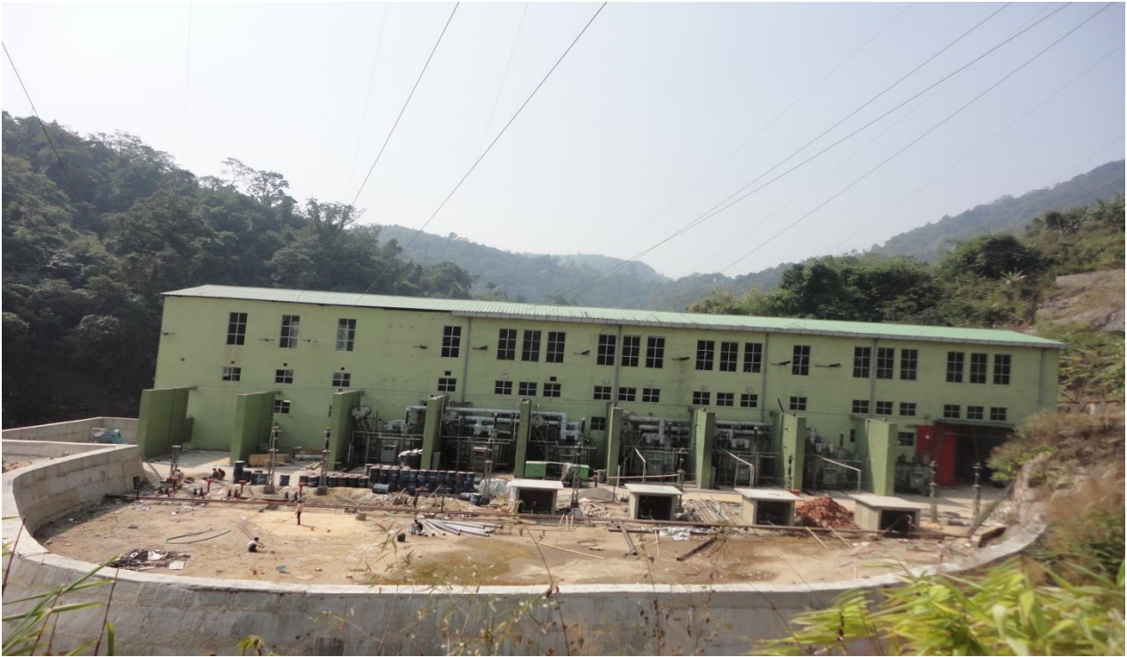
Protection Wall behind the Power House
