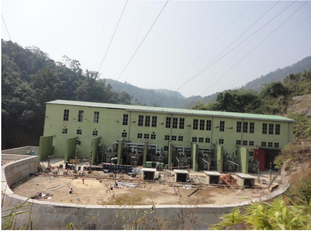
Fig: Protection Wall behind the Power House
