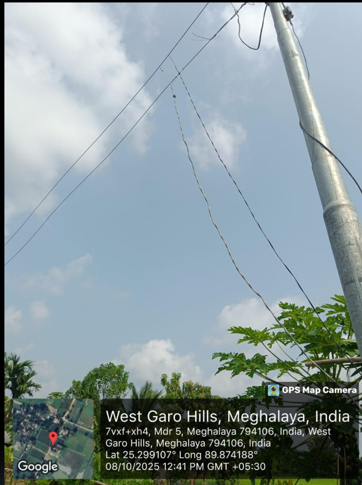
Direct hooking from low tension line.
